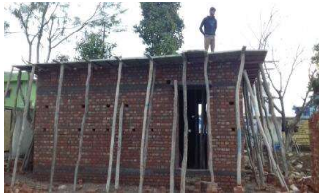
Under construction in Badowala
